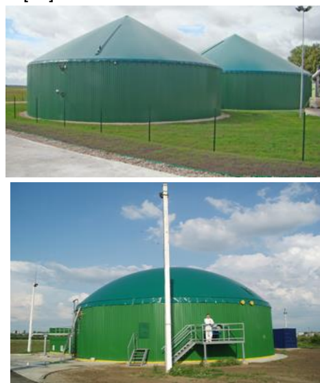
Figure 1 - General view of the production lines for the extraction of biogas
