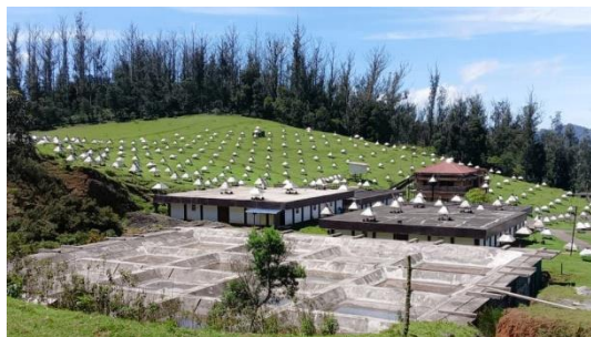
Figure 6 A view of the present-day GRAPES-3 experimental site. The new muon station is located nearby in a single hall. The old muon stations, situated a bit farther away in four different halls, use the similar KGF counters built more than a quarter-century ago.
