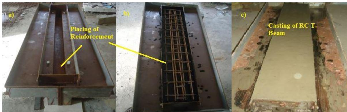
Figure 2. Placing of Reinforcement in T-Beam Steel Mould and Casting of Reinforced Concrete T-Beam
