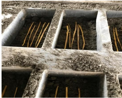
3d) Placing Rice- straw in Layers
