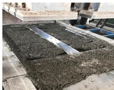
3c) Placing of materials
